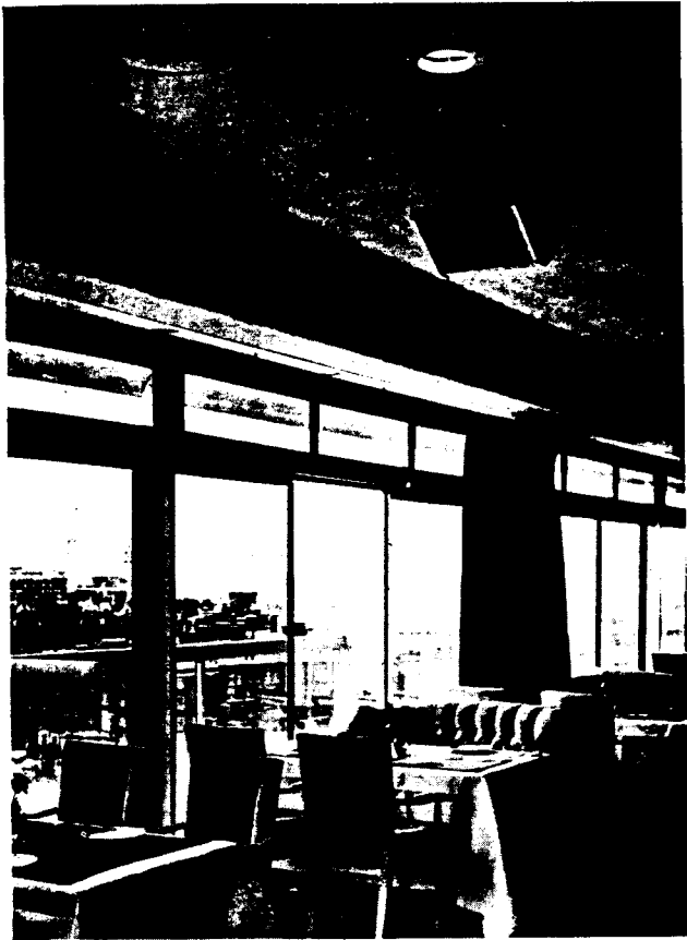
Fig. 1. Roof restaurant at Royal Garden Hotel, showing one of the bidirectional loudspeakers fixed to the ceiling in place of units behind the circular grilles in the ceiling.
