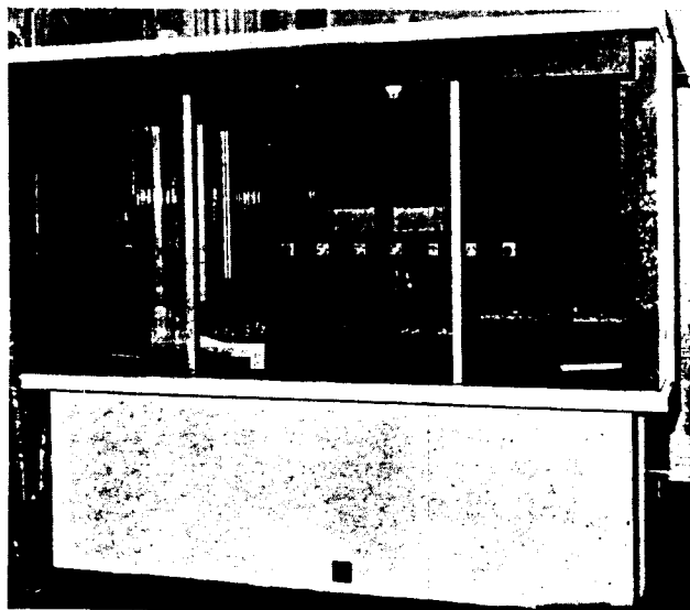
Fig. 11. Inside the control booth for the ballroom, showing loudspeaker switching panel (left), control desk (center), and microphone jumper panel (right).
